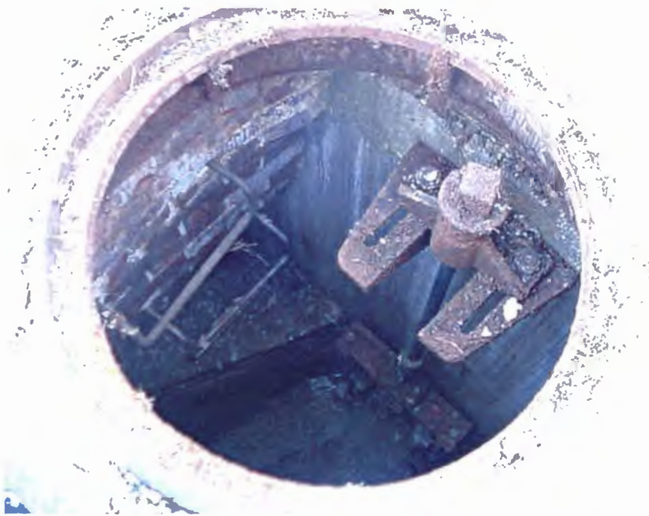
Figure 2-3. Sluice gate at Farmington Road CSO Regulator (003)
