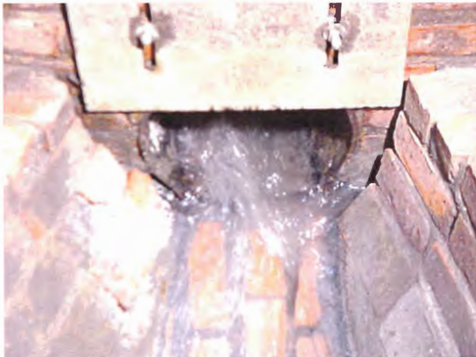
Figure 2-10. Plate on dry weather connection at Lock Street CSO (009)
