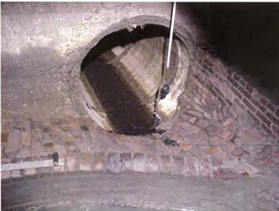
Figure 2-6. Weir and overflow pipe at East Hollis Street CSO Regulator (005)
