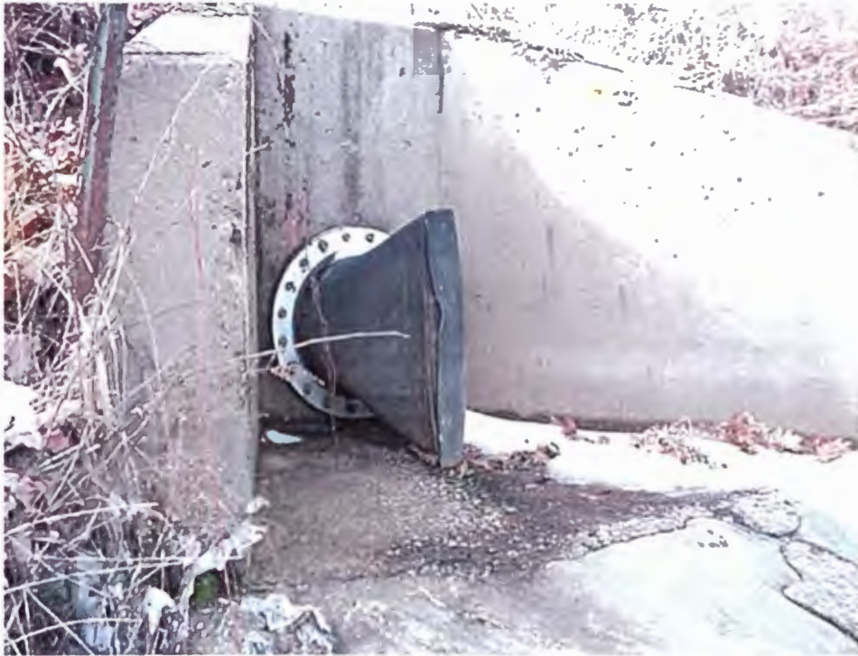
Figure 3-4. "Duckbill" type valve on overflow at Burke Street CSO (004)
