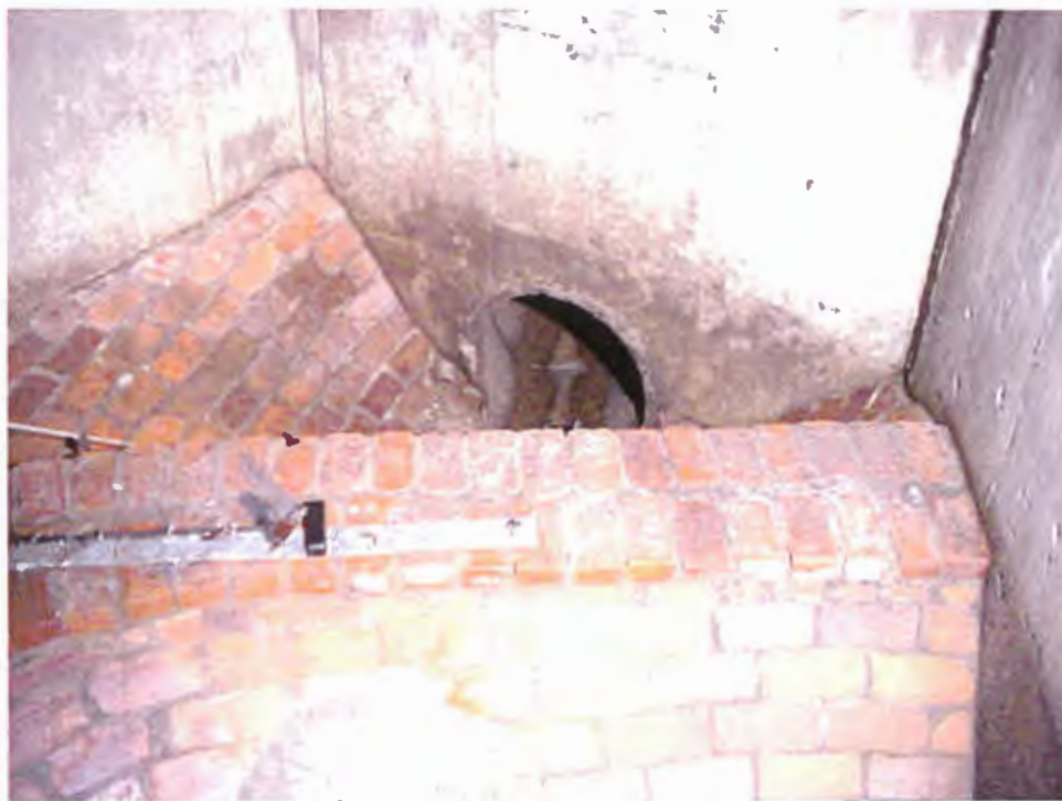
Figure 2-4. Weir and overflow pipe at Burke Street CSO Regulator (004)
