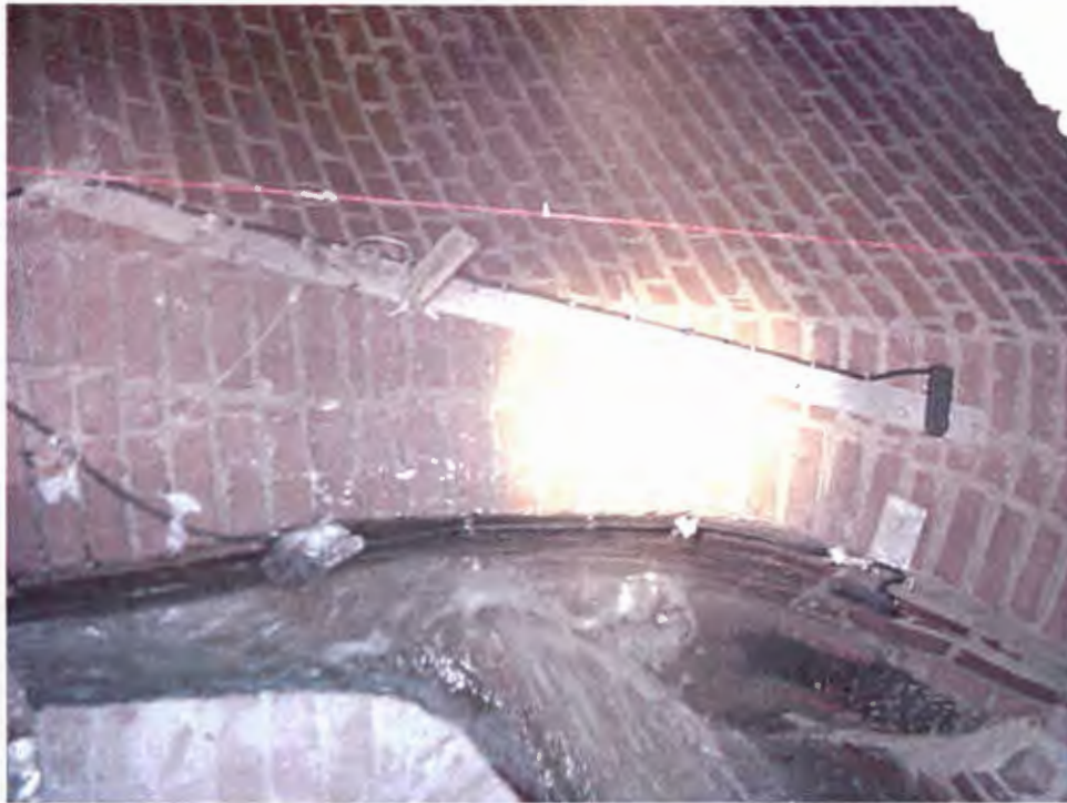
Figure 2-9. High velocity influent flow and overflow weir at Broad Street CSO structure (008)
