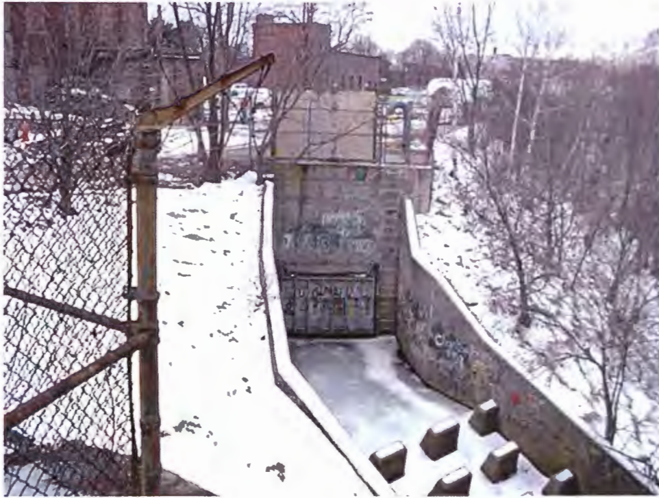
Figure 2-7. Spillway and energy dissipaters from Nashua River Overflow (006)
