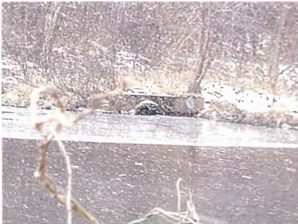
Figure 3-5. Tampa Street CSO outfall partially submerged in Nashua River
